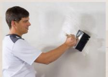
Use a roll for applying a primer coat made of diluted rigid foam adhesive (add 20% water) and let it dry before further processing.
